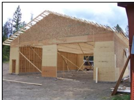
The start of the new building in August 2011
